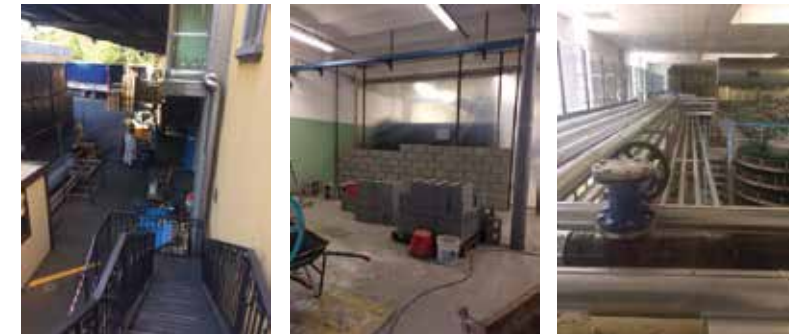
Carlsberg - The interventions for the realization of the pasteurizer
